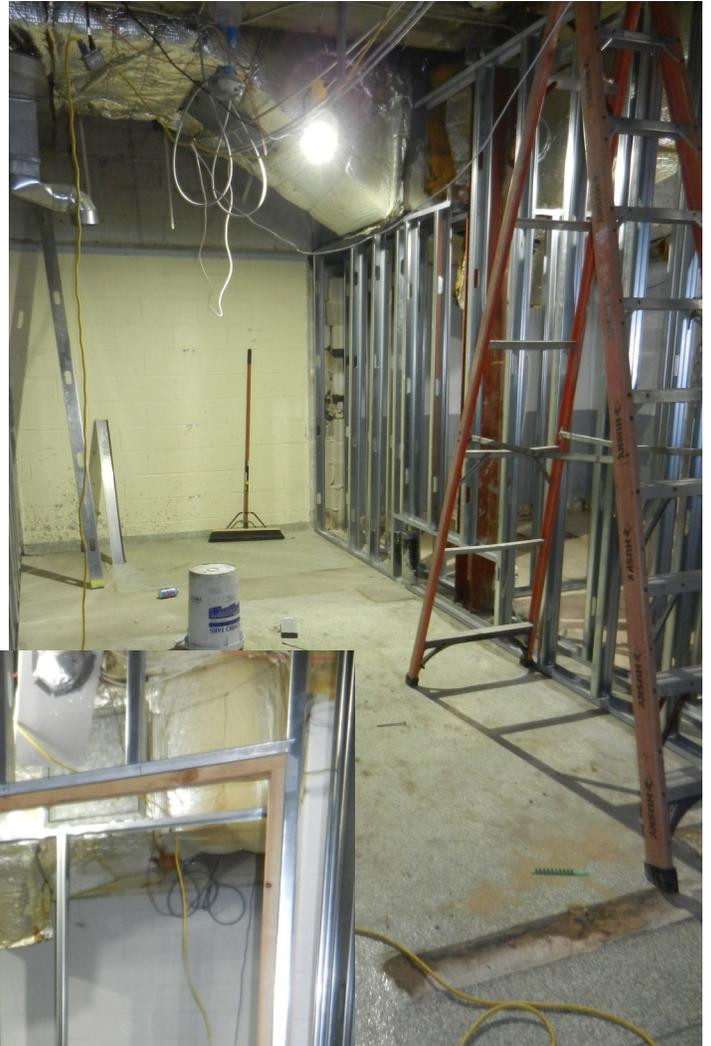
The floor has been filled with concrete and the wall studs are going up. Above is the Men's Room looking out toward the Auditorium. To the right is the front ADA Restroom looking back toward the second restroom in the former dish washing area..
