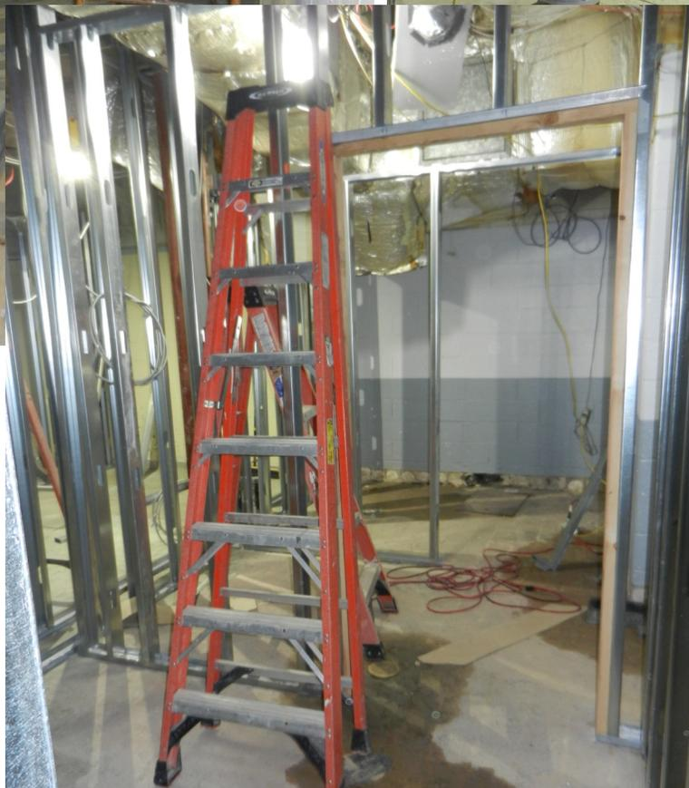
Above is the Ladies Room looking from the doorway, now 4 feet deeper. Note the steel beam that was in the wall between the Ladies Room and the dishwashing area. The foreground shows the indent from the old front wall.
