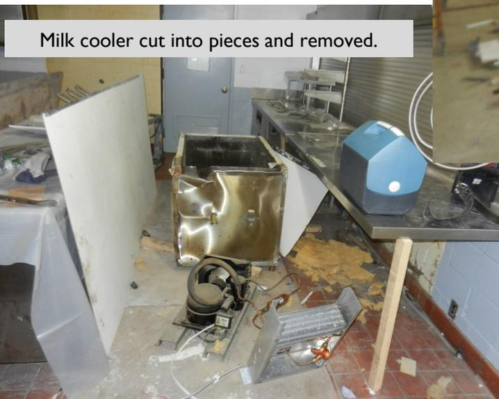
Milk cooler cut into pieces and removed.
