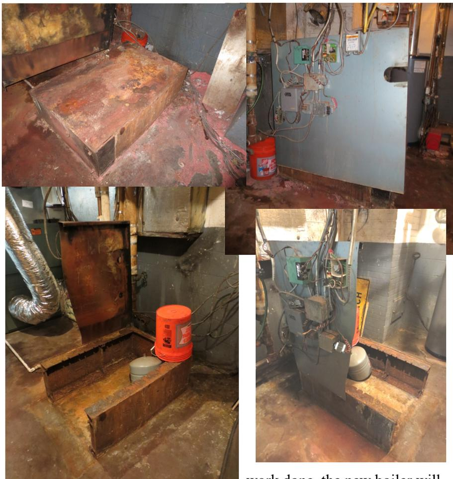
The work continues in the Parish Center for our new furnace. As you can see in the photos above, the panel holding the controls has been modified and the base of the old boiler has been further removed.
