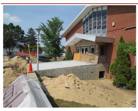
On Monday, the base concrete for the bridge deck was poured over the steel deck. The weather was perfect and there were no problems. As of today (Tuesday) we await the backfilling of the hole where the new sidewalk with wheelchair access will stand (lay?). Installation of the insulation and wirework for the for the ice melting system should be evident as you attend today.
